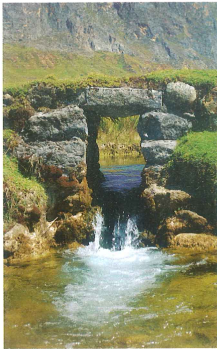
One Inca bridge type consisted of a flat stone placed over a stone-lined culvert, above. In agricultural areas, the Incas often erected 1 to 2 m high walls on both sides of the road to separate it from their crops, below. The walls were made of stone or sandy clay depending on the materials available.
