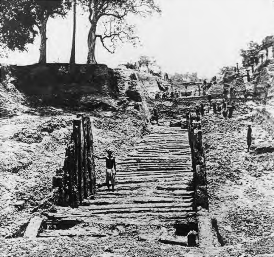
Archaeological excavations have unearthed parts of the defensive palisade, constructed of timbers almost 5 meters (16 feet) tall, that surrounded Pataliputra during Mauryan times.
