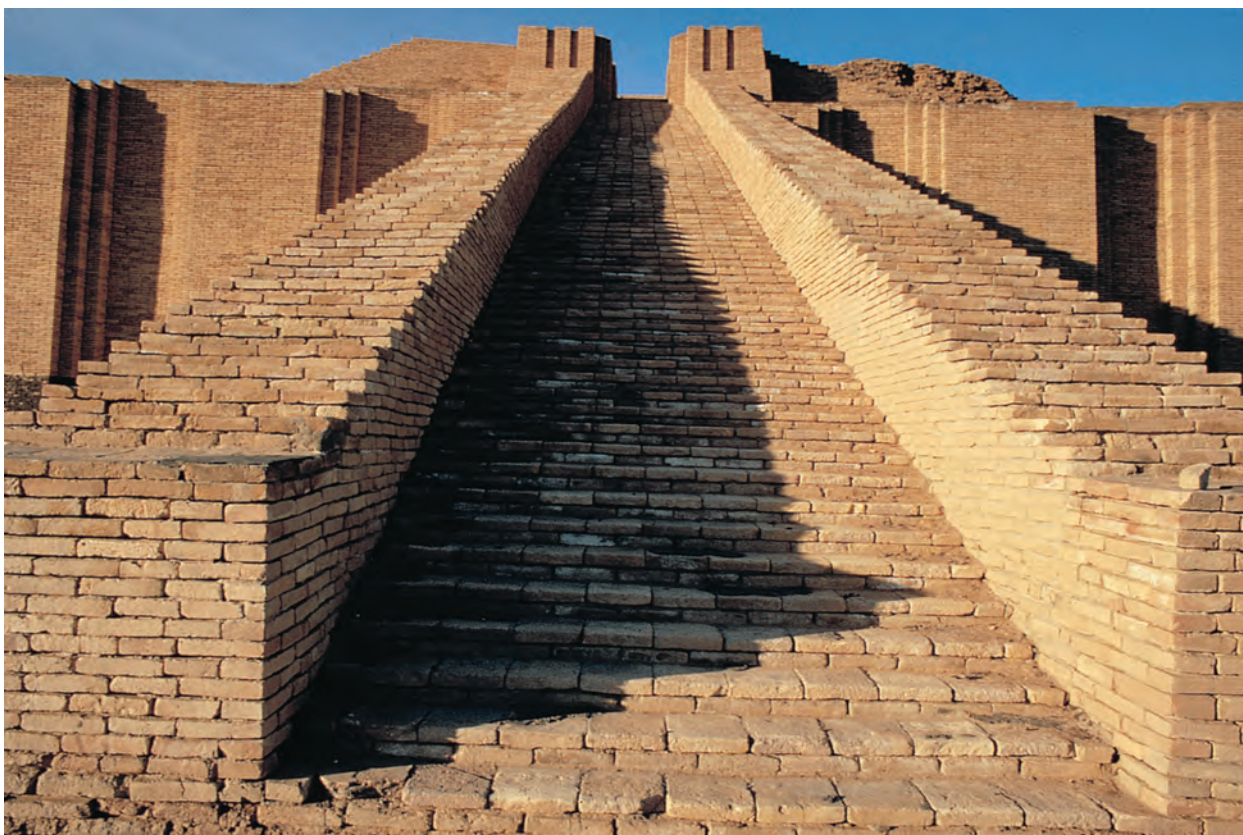
The massive temple of the moon god Nanna-Suen (sometimes known as Sin) dominated the Sumerian city of Ur. Constructing temples of this size required a huge investment of resources and thousands of laborers.
